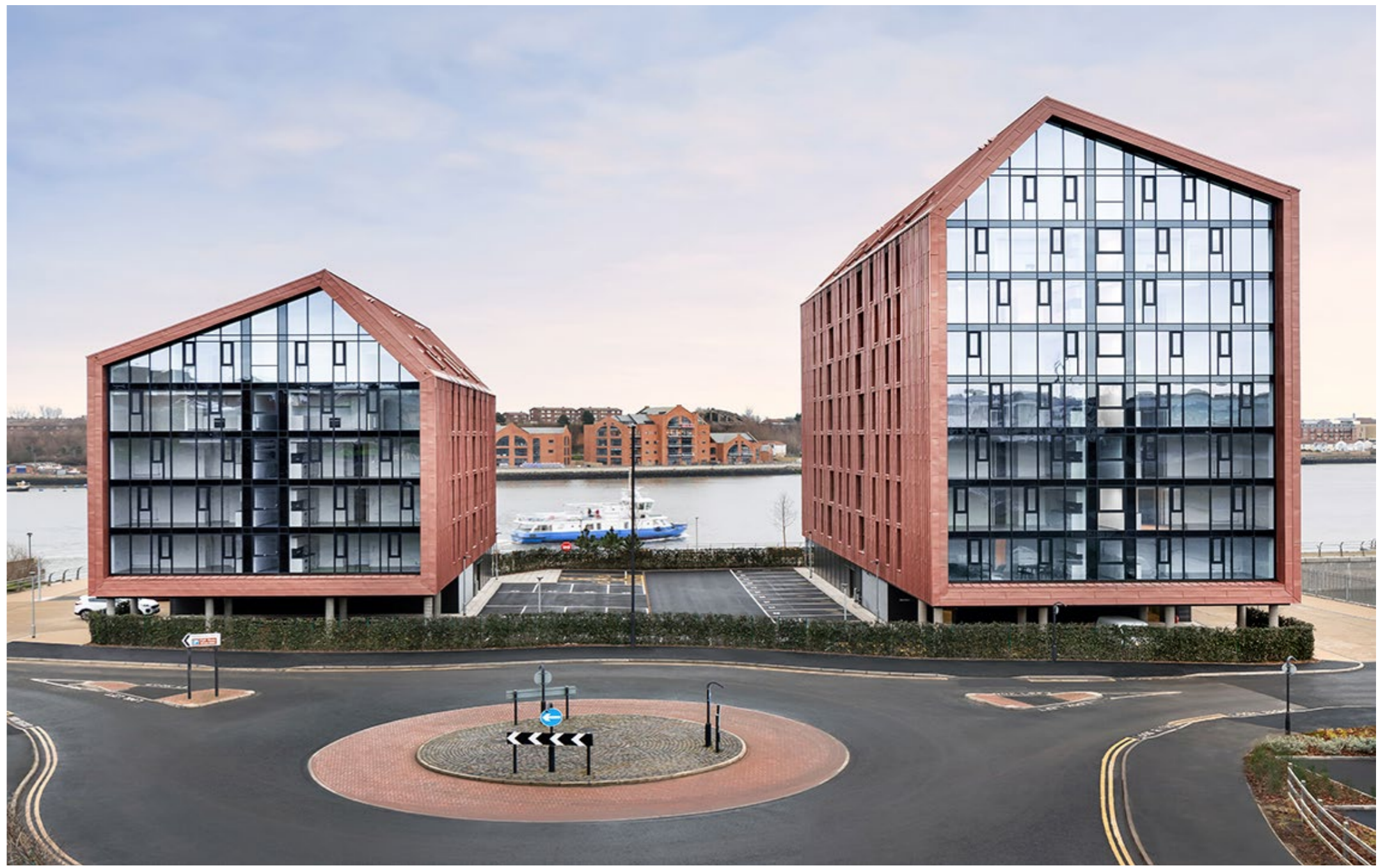
Completed Phase 2 - Smokehouses Scheme
