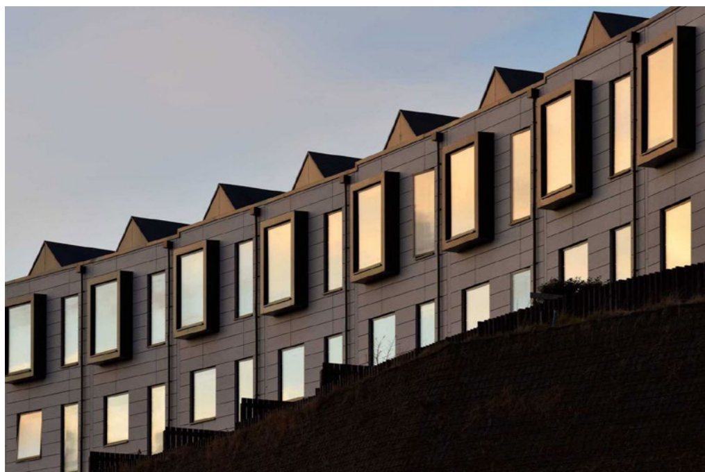
Completed Phase 1 - Townhouses
